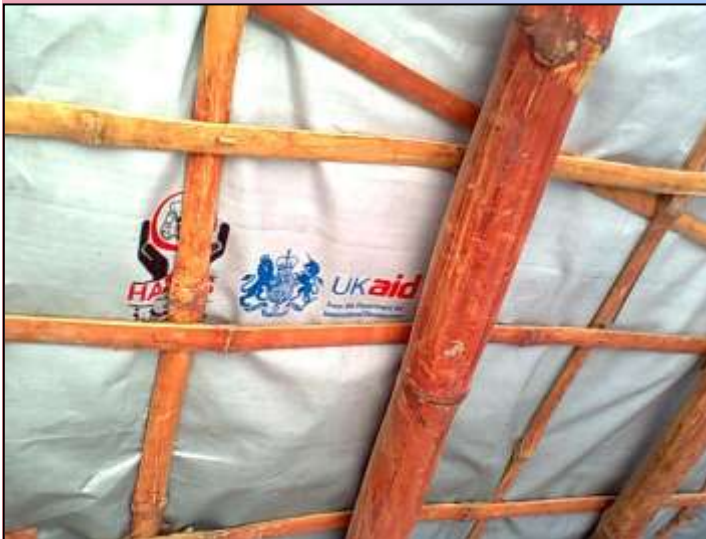
Roofing kits provided to the beneficiaries
