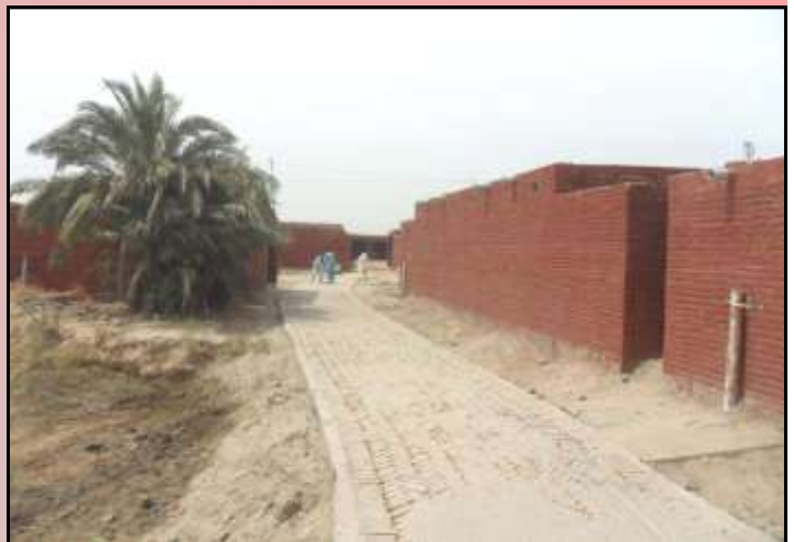
Construction of pavements and one room shelter
